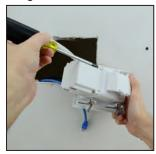
Now screw the white old work box to the back of the bottom plate.
