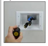
Using a Phillips screwdriver, tighten the screws with wings. These wings fasten tightly against the back of the wall. **Note:** Do not overtighten screws.
