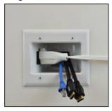
Now hang your flat panel TV on the mounting bracket (not included) and plug your TV into the top power output plate. Then plug your power cord set into the bottom power input plate. Complete installation by plugging the male end of the power cord set into the nearby wall receptacle.
