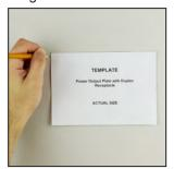
Using the template supplied (see page 5 of instruction sheet), trace the opening for both the top and bottom plate. See Figure 1 before tracing your opening. Remember, the plates are designed to be mounted centered between the studs. Using a drywall saw, cut a hole in the drywall the size of each template.
