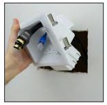
After inserting your low voltage cables and the electrical building wire through the opening for the top plate, insert the top plate into the wall by inserting the electrical work box into the wall first (see Figure 4).
