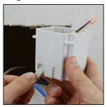
Now that you have pulled the top power outlet plate's electrical building wire though the bottom hole, bend the wire straight. Push the stripped end of the wire through the opening in the white old work box.
