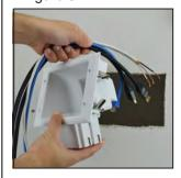
Run your low voltage cables and the included 14/2 with ground UL approved electrical building wire from the top opening in the wall through the bottom opening in the wall. You will need to fish the cables from the top opening to the bottom opening.
