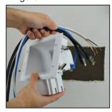
Insert the stripped end of the wires into the push-in connectors. First, insert the stripped black wire into the open side of the push-in connector with the black wire – be sure to push the stripped black wire completely into the connector. Now insert the stripped white wire into the open side of the push-in connector with the white wire. Next, insert the bare copper ground wire into the open side of the push-in connector with the green ground wire.
