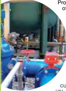
Protecting the pump: detection of no-load operation by undercurrent control, detection of jamming by overcurrent control.
