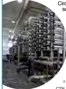
Circulation pumps management, supervision of flow pressure and temperature of osmosis processed water
